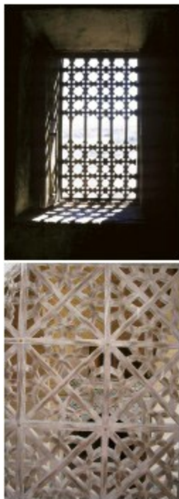
172. Berber wooden grid in a kasbah(fortress) in Agdz, Morocco
