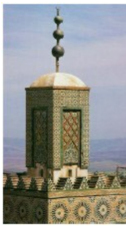
2. Sidi Halaoui minaret, Tlemcen, Morocco
